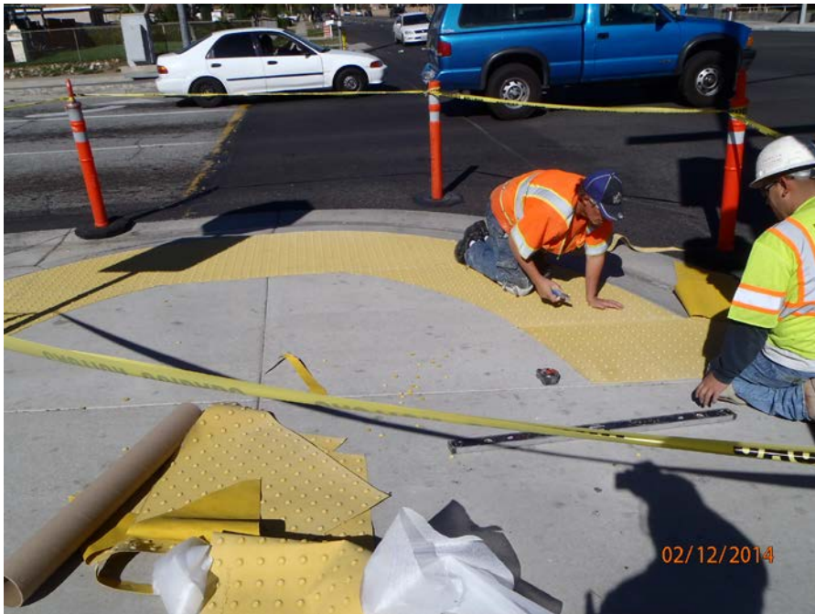
2. Little Mountain and Kendall installation of truncated domes.
