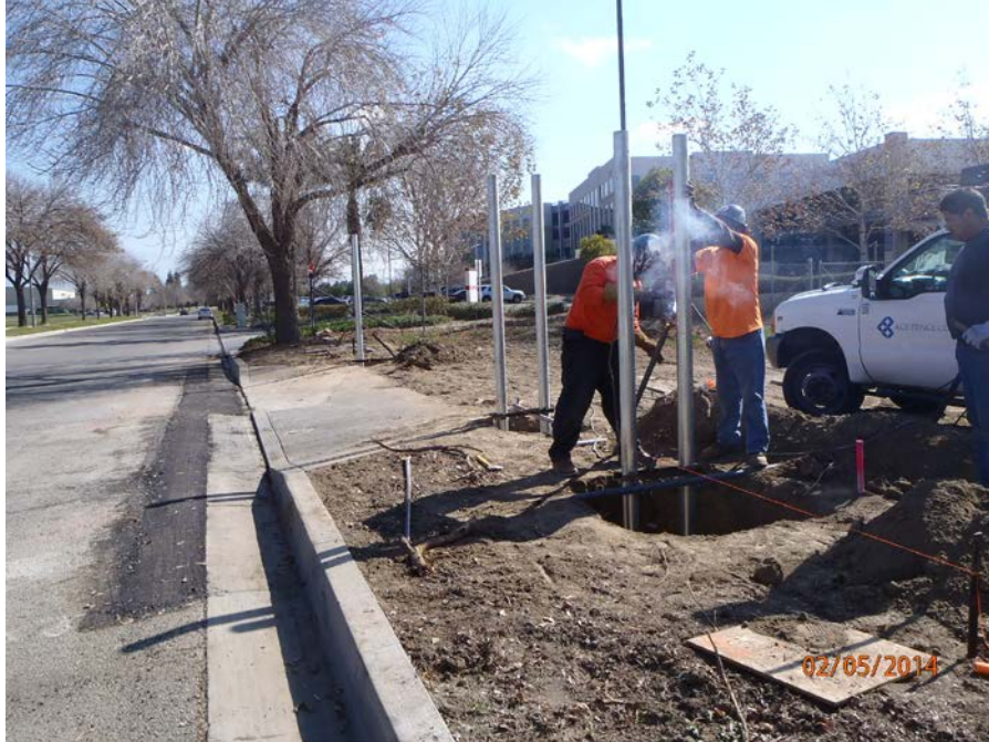
1. Ace Fence installing a gate post for Gage Canal at Brier.
