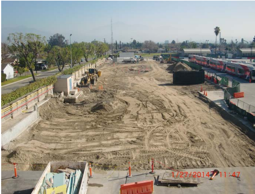
1. Removal of the 600-Gallon Underground Diesel Tank.
