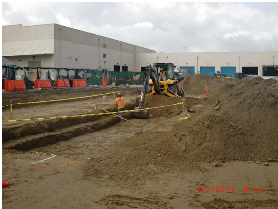
2. Excavating for Building Footings at New Bus Wash Facility (Building B).
