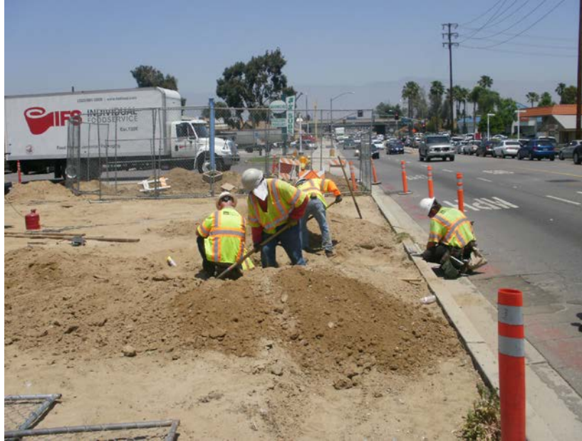
1. Pot holing for utilities at Anderson/Redlands Park-N-Ride in Loma Linda.
