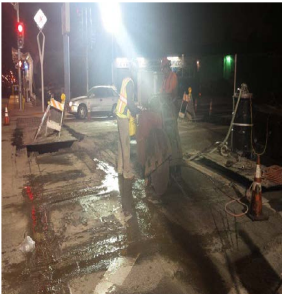
Saw cutting at Baseline Station
