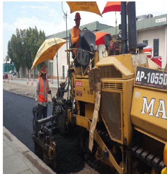
Repaving underway on E Street
